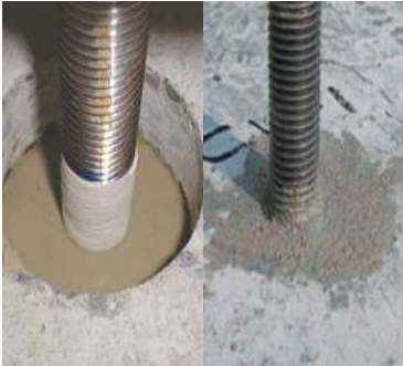
Anchor bolts and bars.
