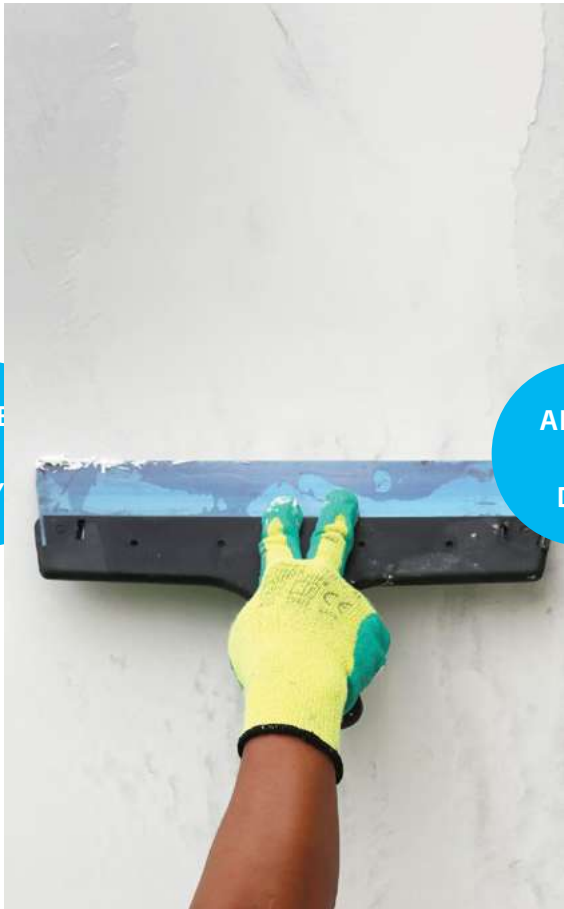
Skim coating (Base coat)
