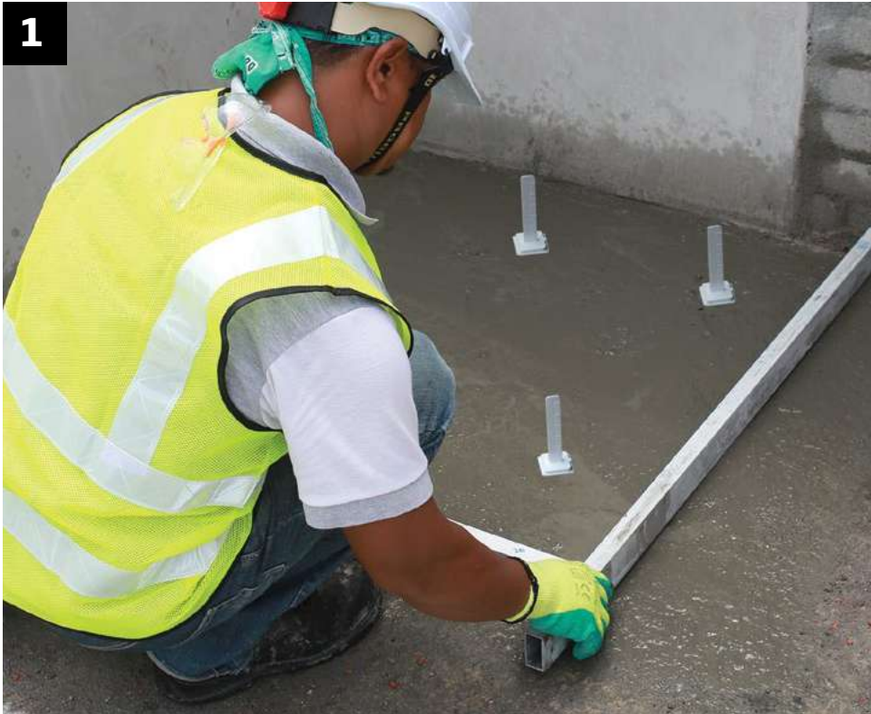
Place level pegs or indicators at regular intervals.
