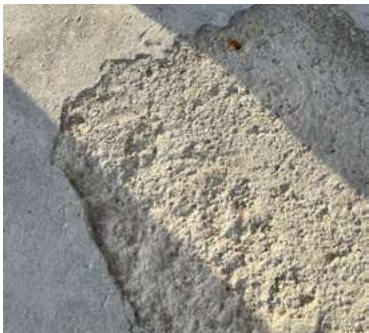
Rectification of concrete surface defect.
