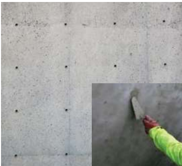
Patching concrete tie-rod holes.
